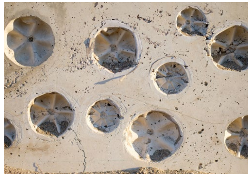
We decorated the formwork panels with the bottoms of plastic bottles, caps and plastic toys. We sorted, cut, arranged, attached, sealed. Thus, after pouring the concrete, negative prints of objects remained in the bench.
