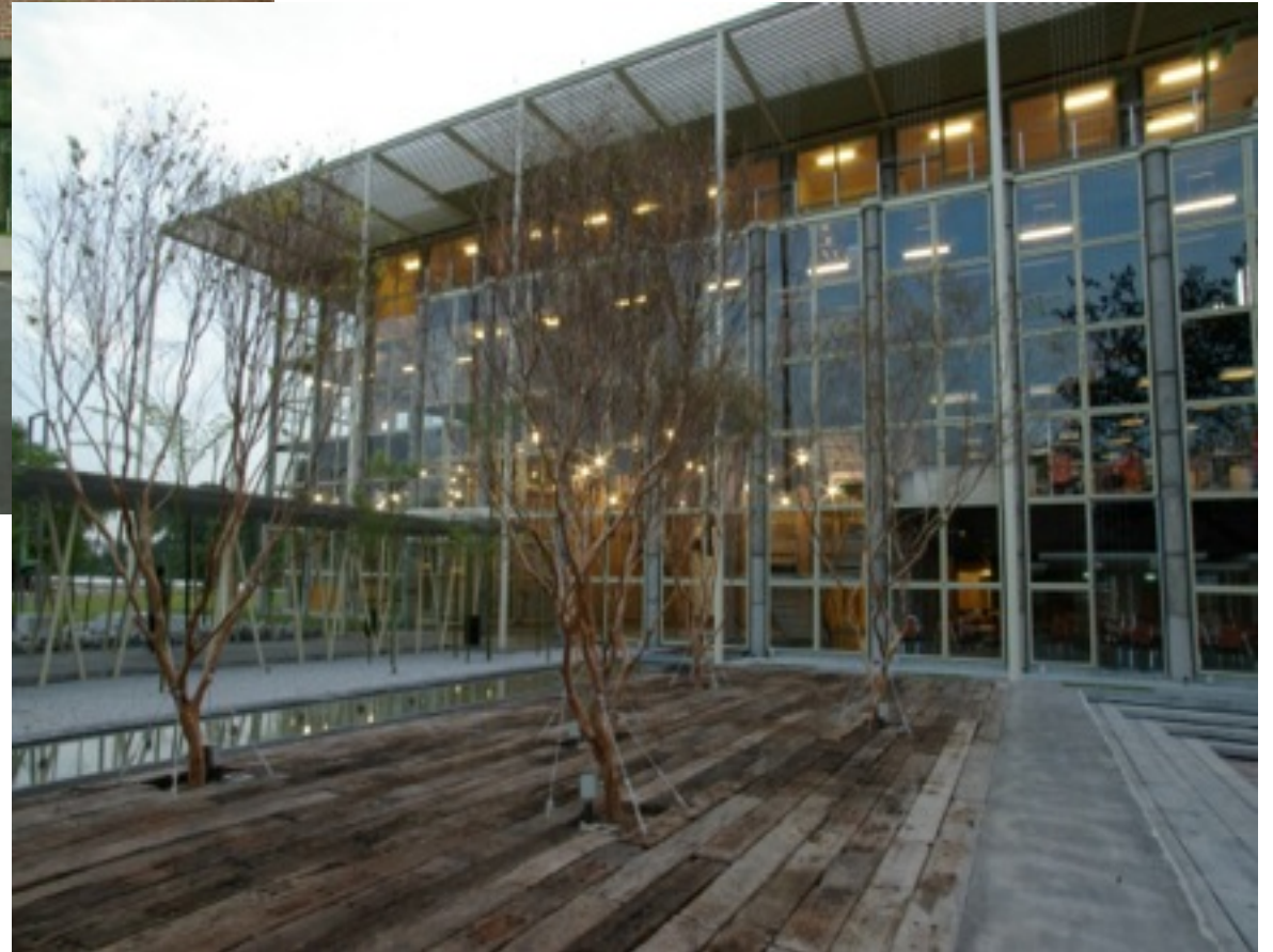
Timeworn railway sleepers reused as part of the landscaping to harmonize the old and new. (below)
